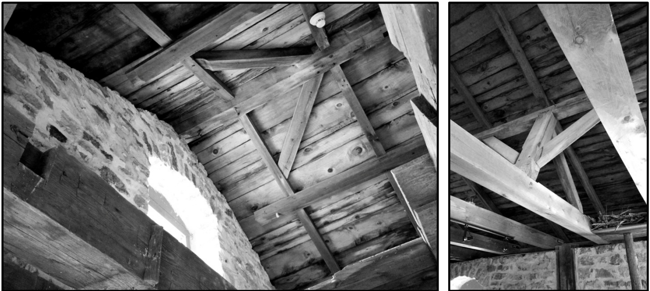
Left: Wind supports (diagonal bracing) on either side of the ridgepole. Right: Queen beam (angled post support of the purlin (horizontal roof support beam)).
